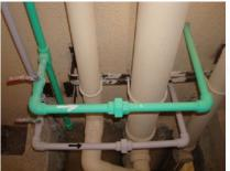
Pipe colour coding and arrow marking.
